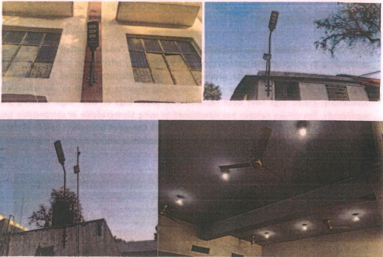
Installation of Solar lights and LEDs at MIER College
